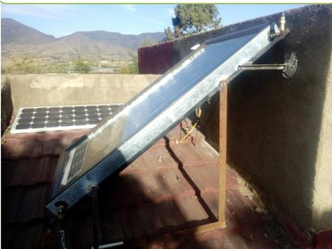
Due to lack of reticulated water, the low pressure pump system uses 50L cold-water storage tank on top to drive the hot water from the 50L geyser underneath
